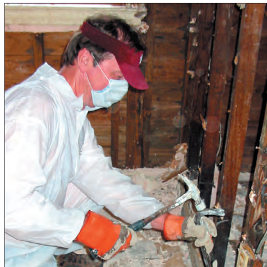
Gerry Trennepohl strips frame of moldy drywall and insulation.
