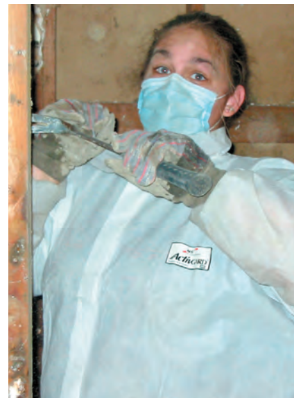
Andrea Dunn removes damaged portions of wall. [Photos by Danney Richardson]
